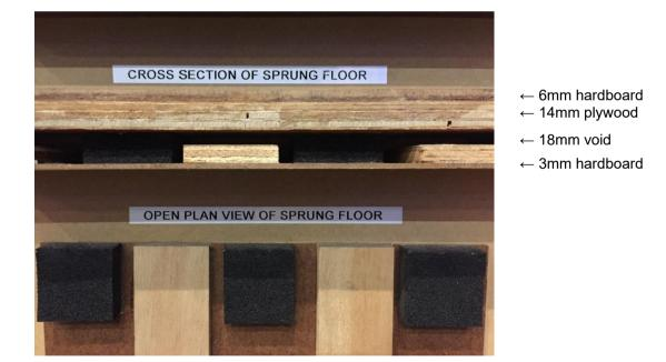
Screwing into the floor can cause significant damage to the top level and subsequent levels, and due to the void/neoprene foam and the thin hardboard at the bottom of each panel of sprung floor, it is not a secure base for anything that may require substantial anchoring. A load under pressure has the potential to cause significant damage.
